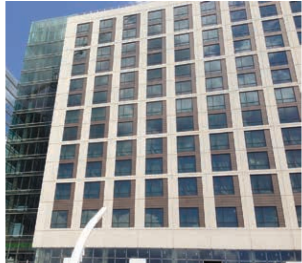
Figure 1a Hyatt Regency expansion, Tysons Corner, McClean, Va. All figures and photos: RTKL Associates.
